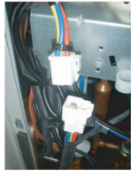
Compressor output terminal joining position
