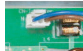
Checking connection between noise filter and inverter PCB power
